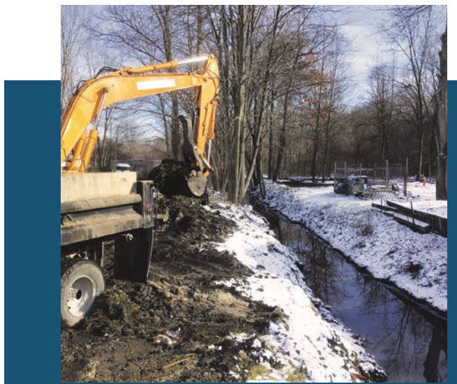
TASD removes debris that was causing water to collect in this ditch and breed mosquitoes.
