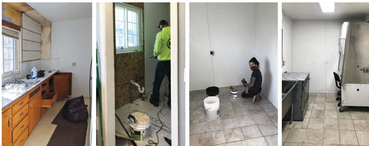
Construction on TASD's Vector-Borne Disease Detection Laboratory.
